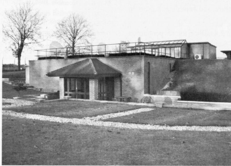
External view of Bunker
